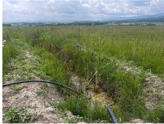
Figure 8: A berm and swale system with a water connection to the uphill reservoir, the trees should provide shade to the cattle in the future.
