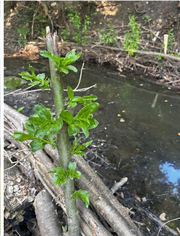
Figure 16: Fascine bundles and living wood will form a permanent natural structure, also providing shade to the river in the future.
